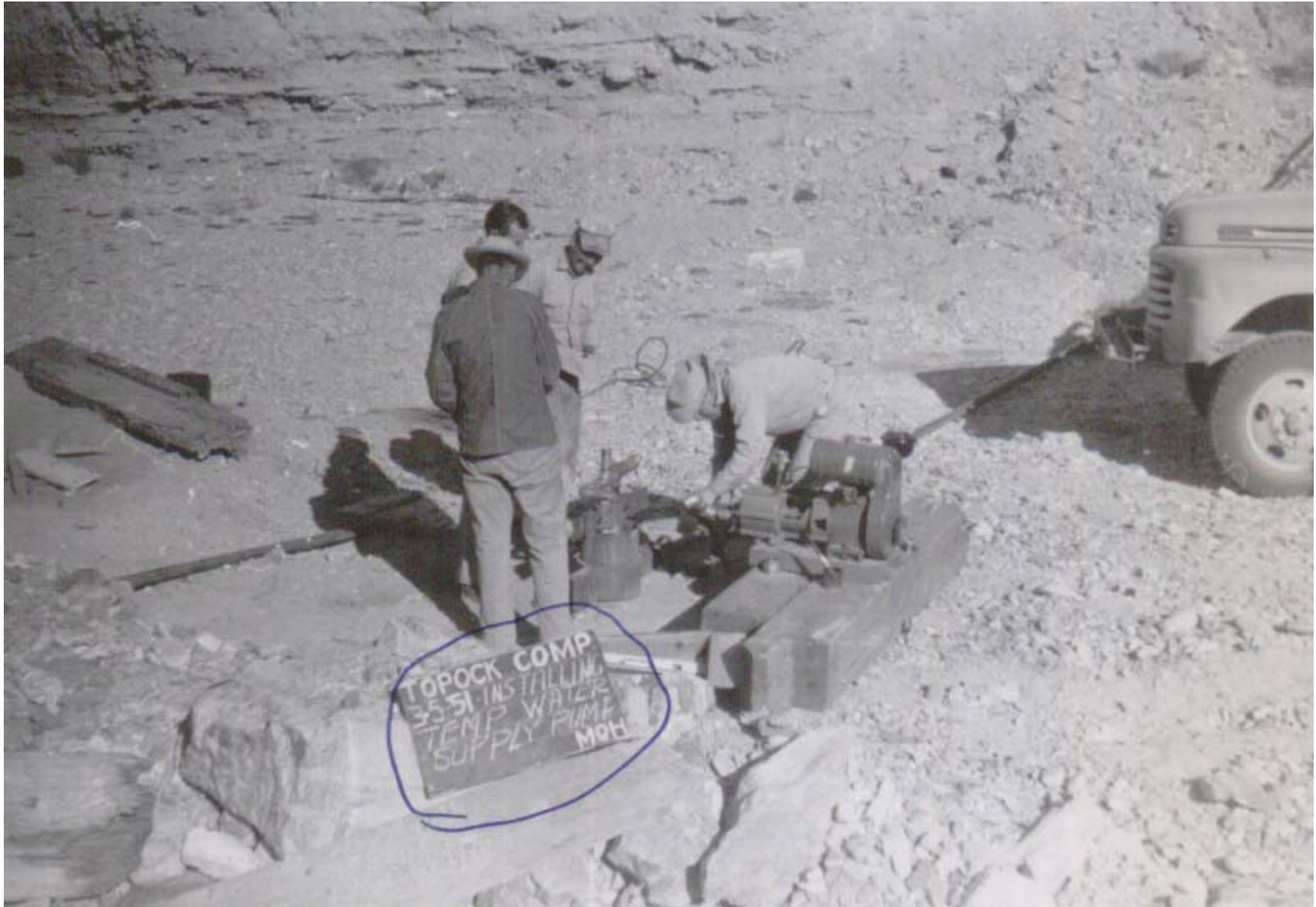
Figure 4. March 5, 1951 Close up of Pump Installation in Temporary Water Supply Well
